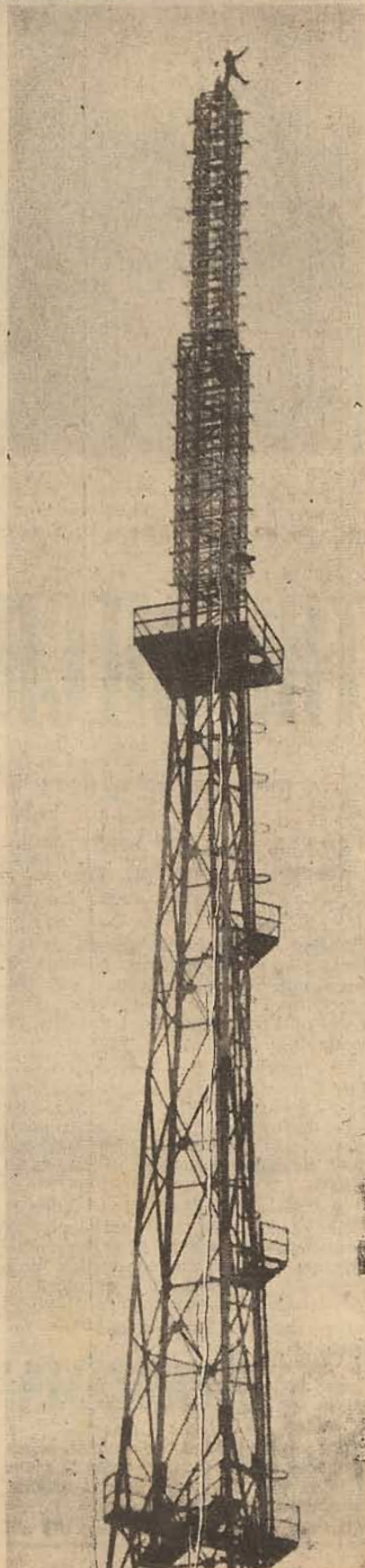
Right—The top of ATN's mast clearly shows the two sections of the aerial itself which commences just above the main platform. The dipoles mounted near their reflectors are clearly visible. The acrobat at the top illustrates by comparison the size of the structure.
