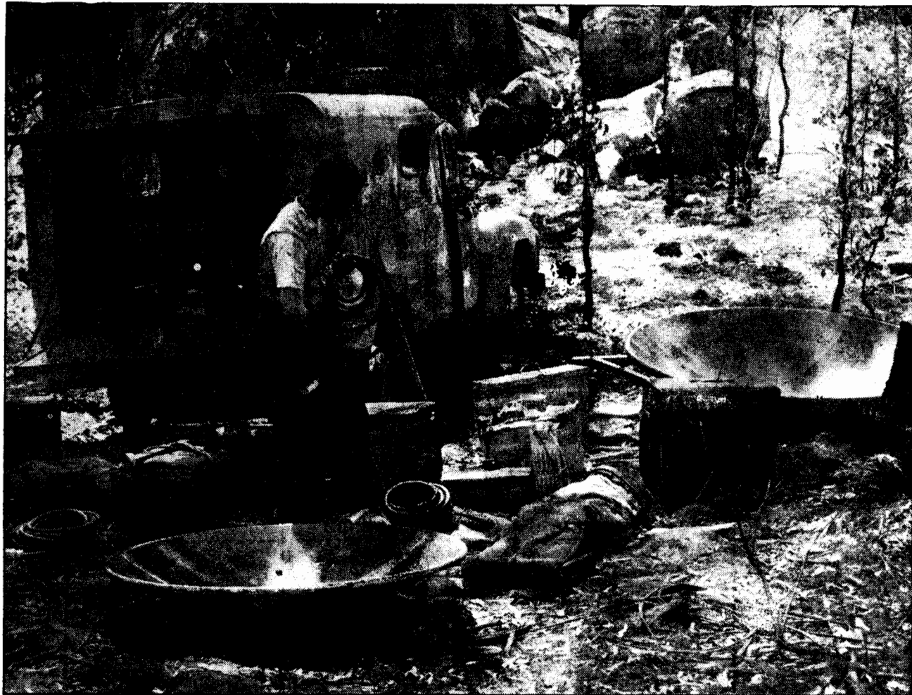
This picture shows the installation at Repeater No. 1 (Mt. Gibraltar). In the back of the van is a motor-generator set for power. In the foreground are seen two of the microwave parabolic aerial reflectors, units of equipment ready to be unpacked, and connecting cables. All this was later manhandled to the elevated site.
